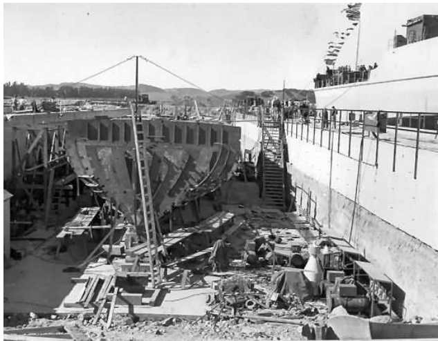
An ARS under construction at Basalt.
