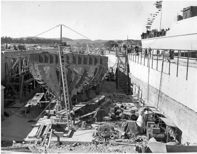
An ARS under construction at Basalt.
